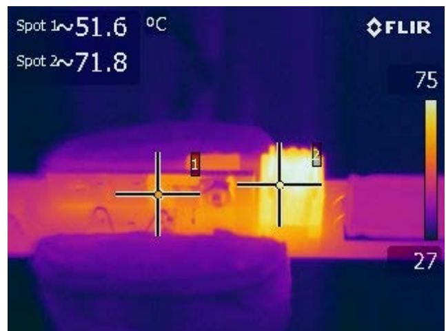
Figure 22 – 265 VAC, Full Load. Spot 1: LYT4213E. Spot 2: Transformer.
