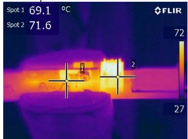
Figure 20 – 115 VAC, Full Load. Spot 1: LYT4213E. Spot 2: Transformer.
